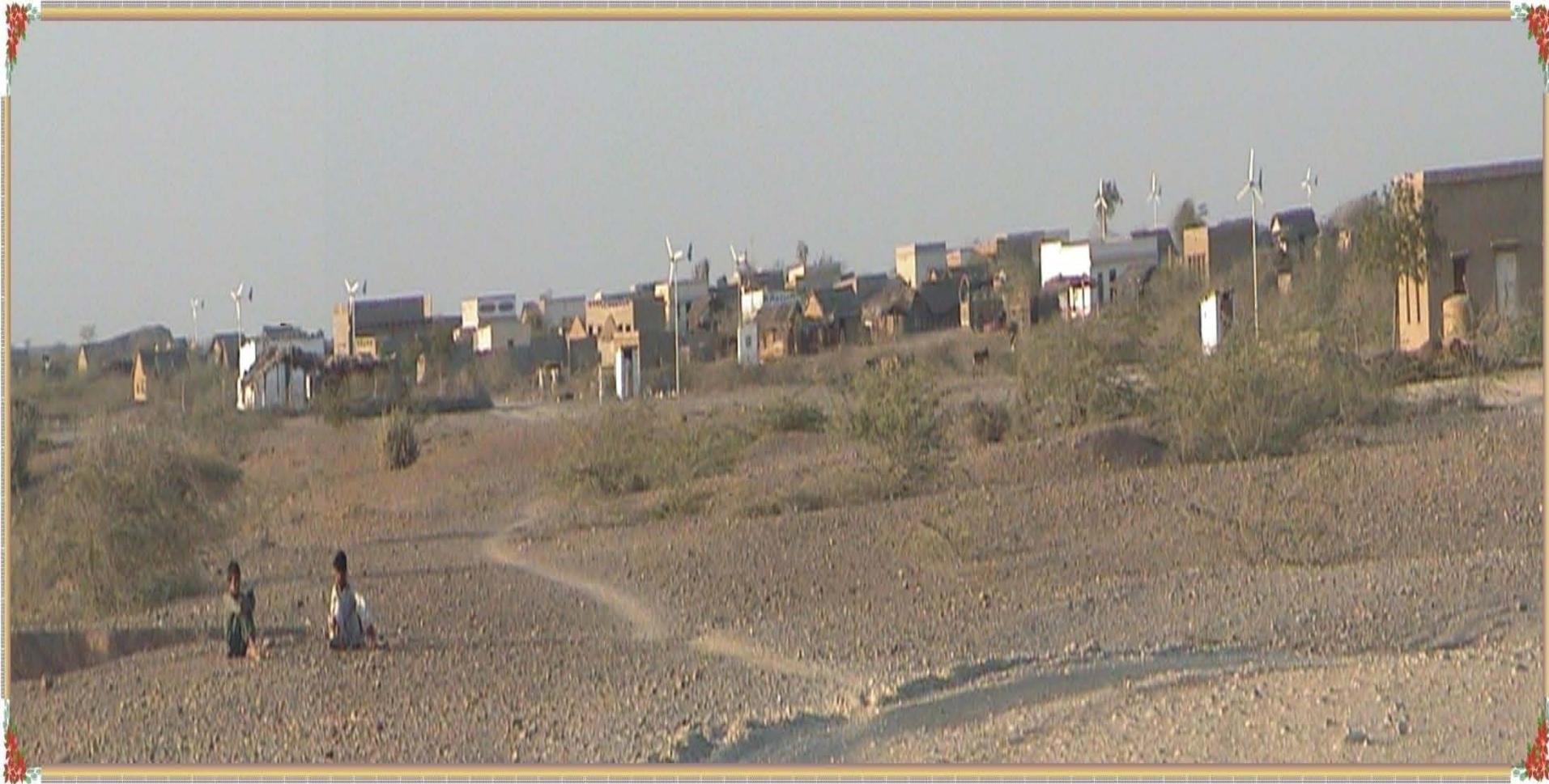
A Panoramic View of Village Gul Muhammad, Showing some of the Wind Turbines installed by PCRET (April 2005)
